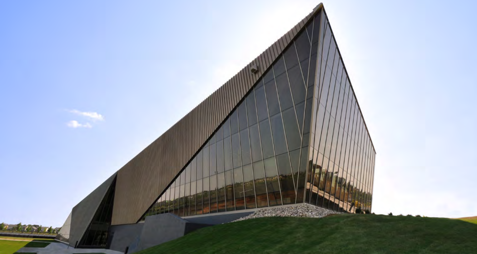
Clareview Community Recreation Centre and Library | Edmonton, AB CISC Alberta Steel Design Award Finalist - Building Communities | 2015
