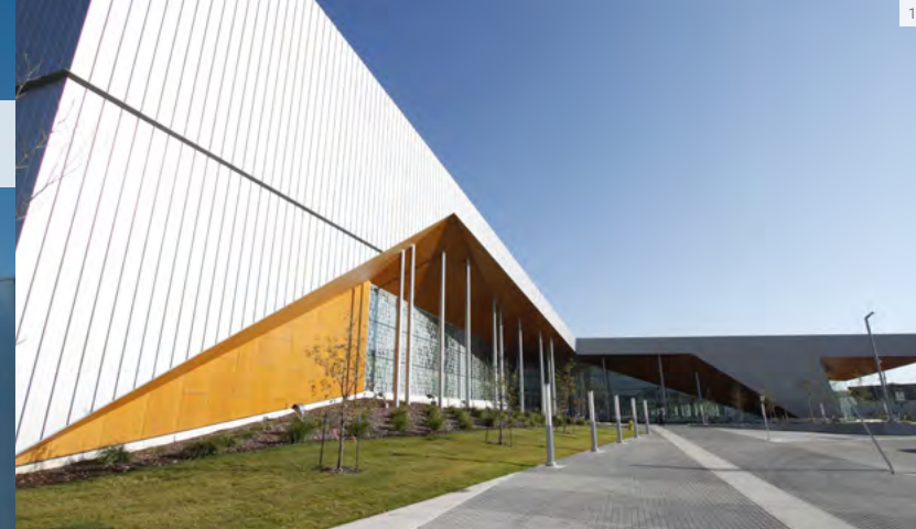
Okanagan College Trades Complex | LEED® Platinum | Kelowna, BC Canadian Green Building Award | Institutional Large | 2019
