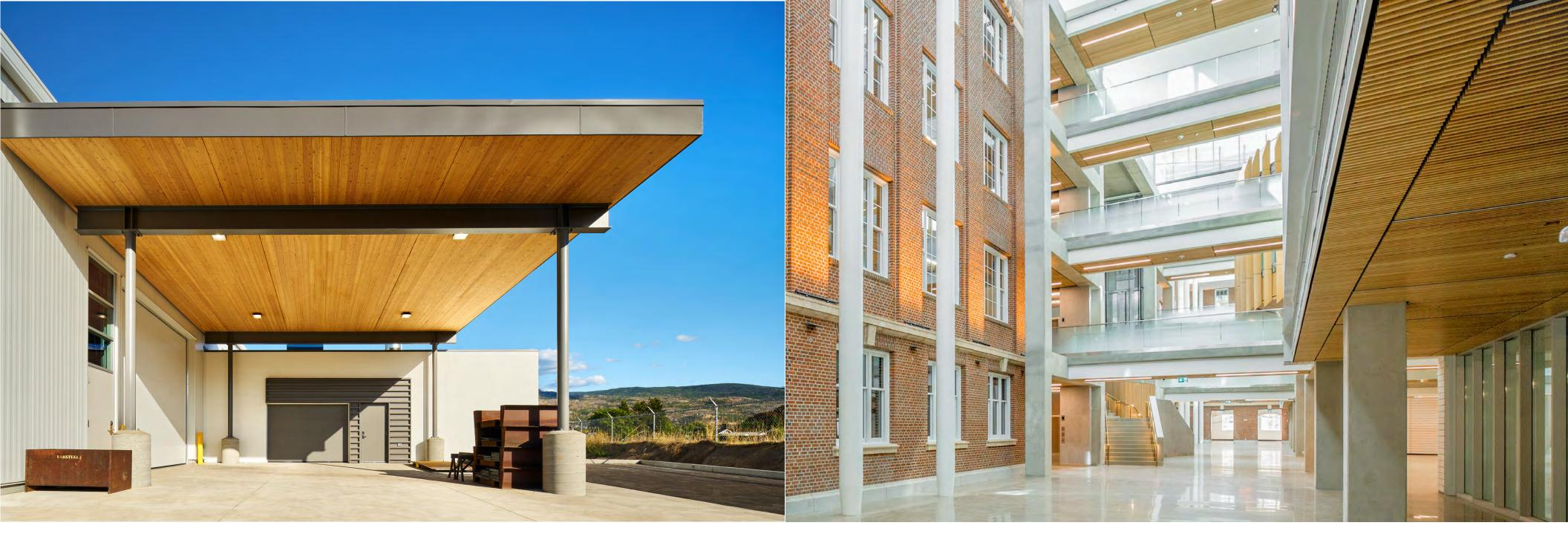
Okanagan College Welding Trades Training Facility Kelowna, BC This project is a one-storey, pre-engineered steel welding facility with canopies constructed from CLT and structural steel. The Okanagan College Penticton Welding building is certified LEED Gold.
