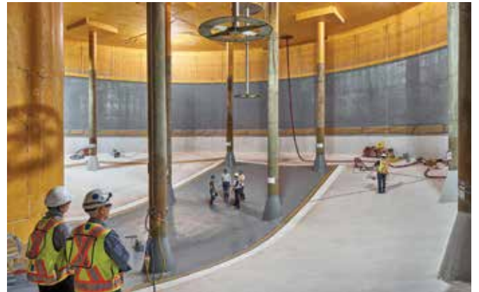
1950s Wastewater Digester Tank, Gold Bar Digester No. 3
