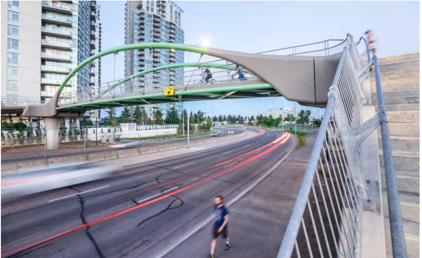
The Westbrook Pedestrian Bridge Overpass, which connects Westbrook mall with the community of Spruce Cliff.
