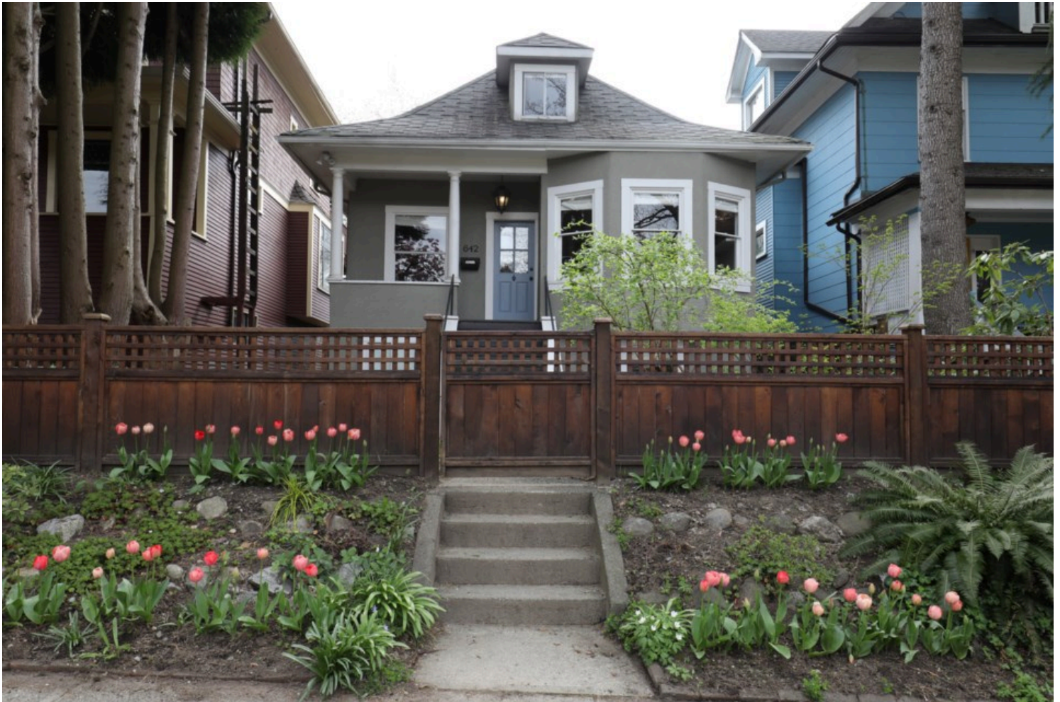
A character home built in 1908 in Vancouver's Mount Pleasant neighbourhood is being reconstructed to net-zero standards, believed to be the first such project in Canada for a house that is 115-plus years old | Photo courtesy of Branden and Sylvie Kotyk
