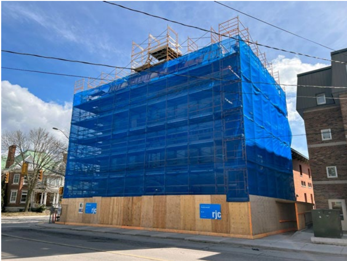
PHOTO COURTESY RJC ENGINEERS – The Bishop’s House under construction in early spring with full height scaffolding to allow access to all areas of each elevation.
