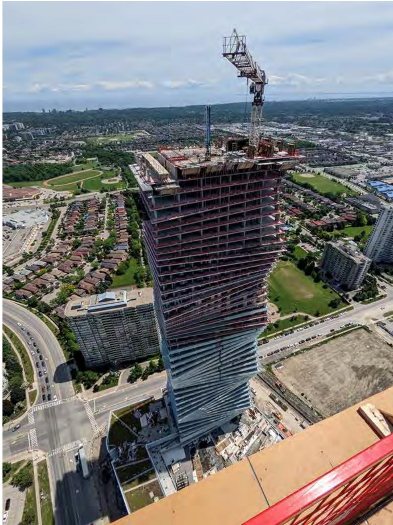
PHOTO COURTESY ELLISDON - A conventional fly form system was used in the construction and the concrete was pumped to each floor, a process that did require some planning and set up time.
