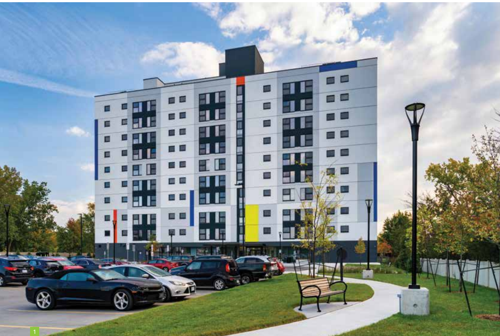
1. The building has a super airtight high R-Value building envelope, triple-glazed windows, thermal bridging mitigation and energy recovery ventilation to achieve Passive House Certification.
