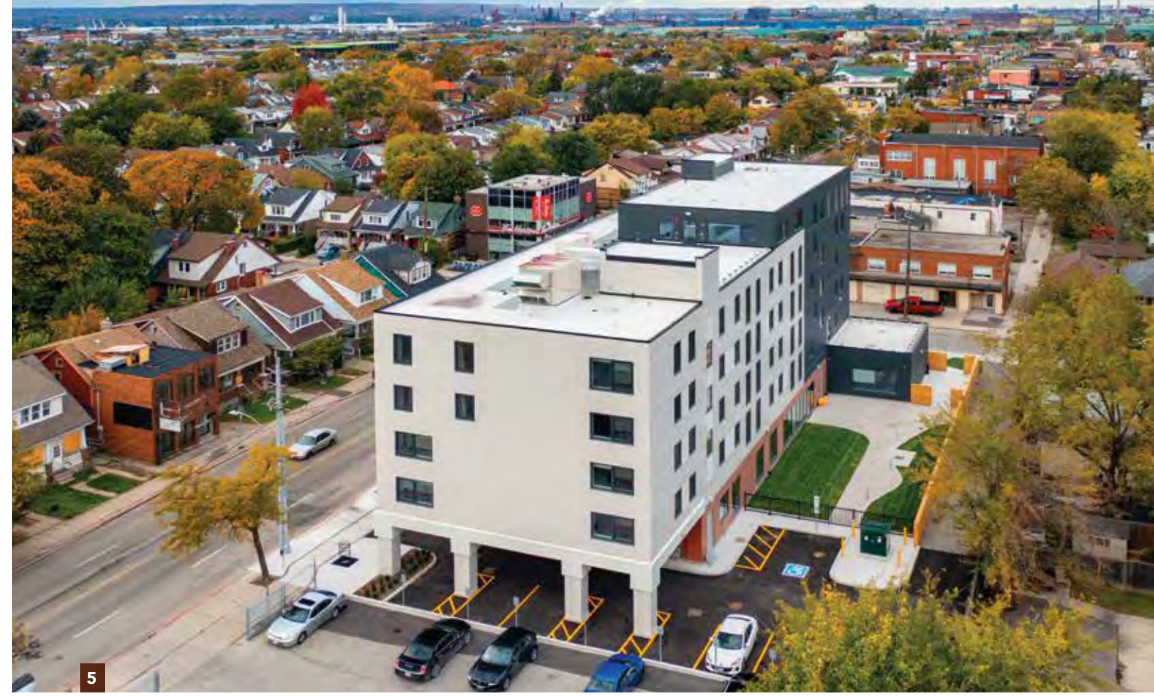
5. The west elevation. The building orientation was determined by the site location, height and program area required. Triple-glazed windows were sized according to their orientation using passive design strategies.
