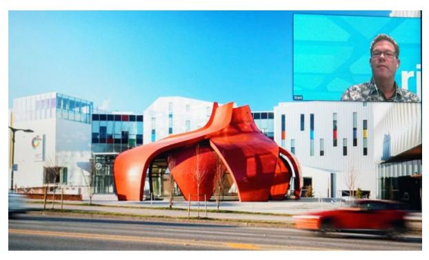
SCREENSHOT — The Great Northern Way Pavilion in Vancouver features curling, overlapping large petal shapes constructed from wood. Its construction was compared to a boat, where there are ribs to help give its shape.
