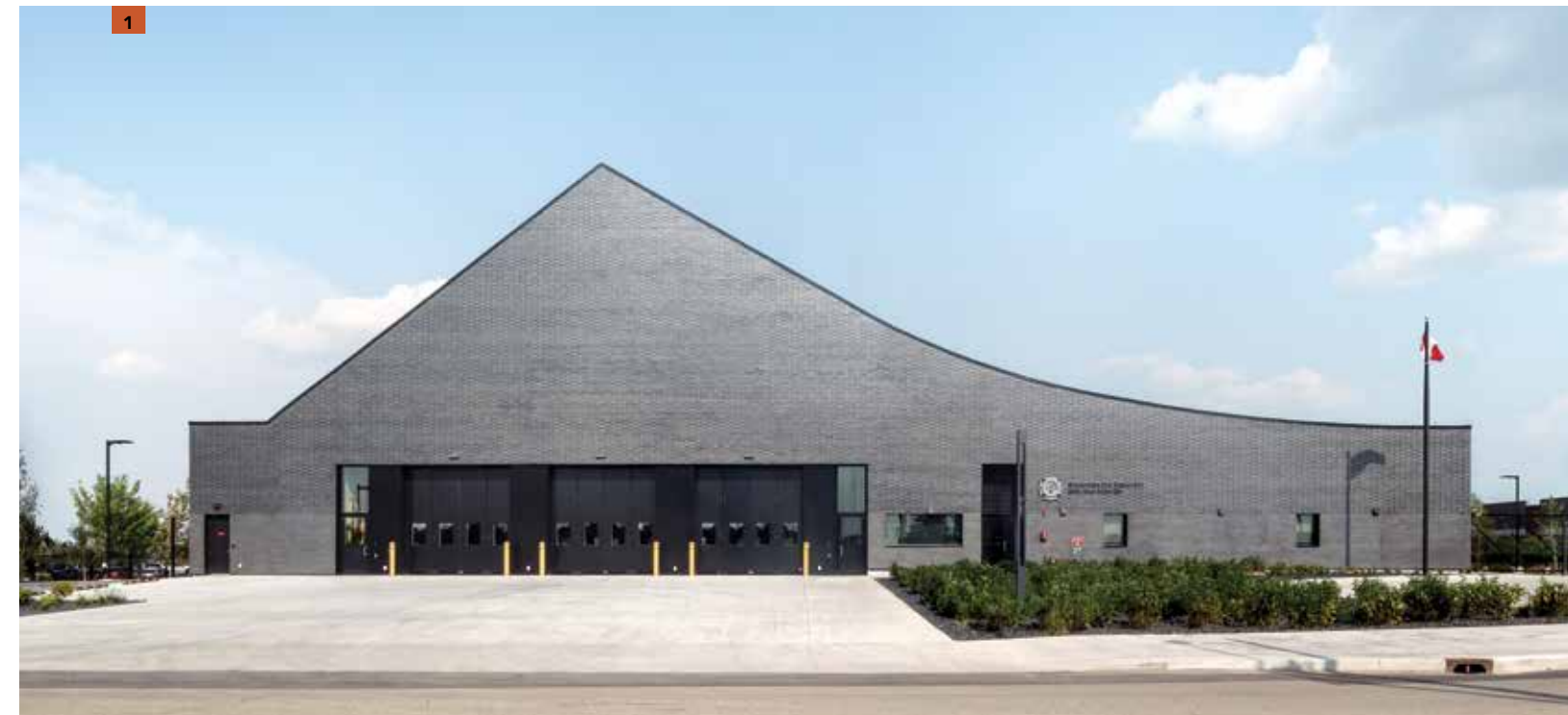
1. The station's distinctive form accommodates a large volume housing the apparatus bay and a smaller volume for the domestic quarters. The overall design conveys feelings of permanence, security, wellbeing, comfort, and longevity.
