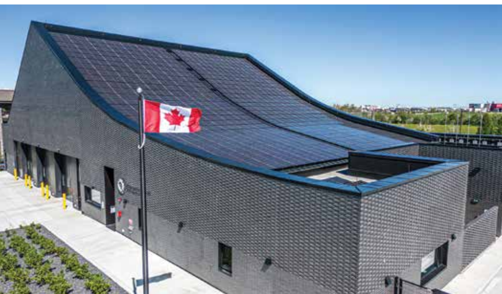
One of the building's key sustainability features is the bi-folding doors that allow the trucks in and out.
