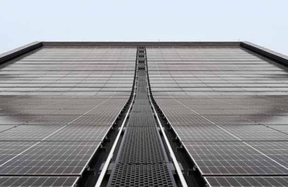
The striking south-facing roof, featuring 382 panels with a rated capacity of 143 kilowatts, is gently sloped to capture the sun's rays most effectively.
