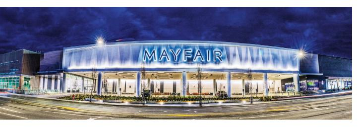
architectural metal panels, glass storefronts, EIFS, and architectural precast concrete panels, built off-site and then trucked in. "We also used cast-in-place concrete for some structural components such as shear walls, pile caps, grade beams, parkade ramps and vertical circulation cores, which were completed by PCL," says Enriquez.
