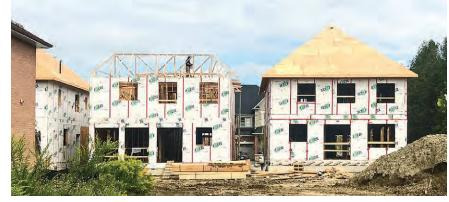
Excel Exterior Structural, Continuously Insulated Sheathing.
