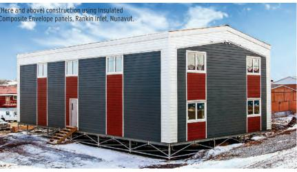
and turn on the heat. Due to the nature of our ICE Panels with their built-in insulation and vapour barrier, once the building is erected and windows and doors are installed, the heat can be turned on and construction can continue.
