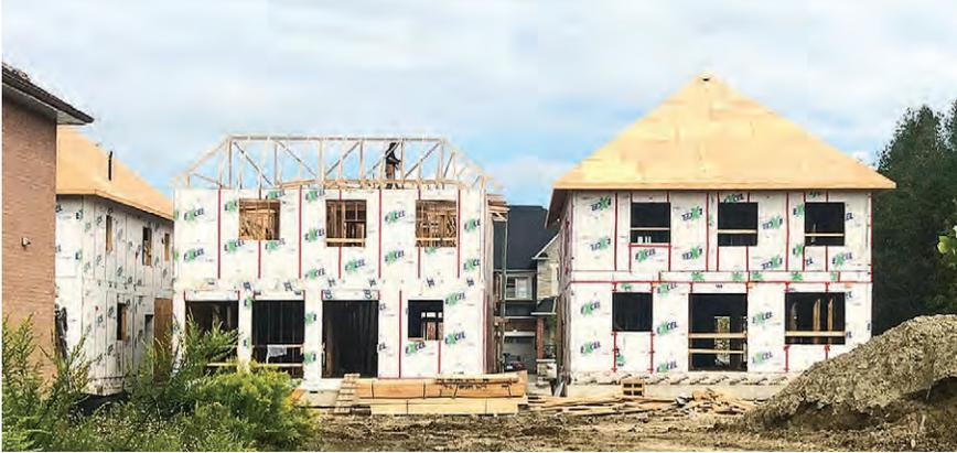
Excel Exterior Structural, Continuously Insulated Sheathing.
