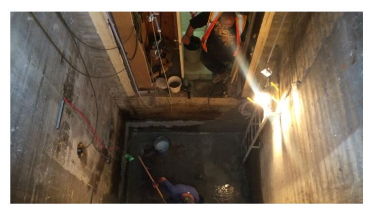
Also, there are lots of bolt holes and anchor spots you can't remove because doing so would mean removing the entire elevator. You then have to work around those by using sealants or other urethane-compatible products to try to trap that water.
