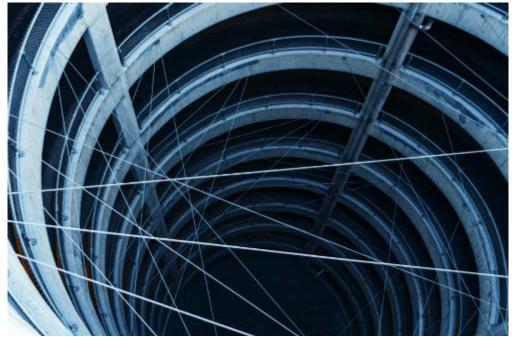
The second design concept, the Descending Spiral, is an installation of crisscrossing cables descending the parking structure's central ramp in a repeating spiral pattern. Again, while seen by many as an artistic element, its actual purpose is to discourage jumpers by changing their perception of a potential free fall from the top deck.
