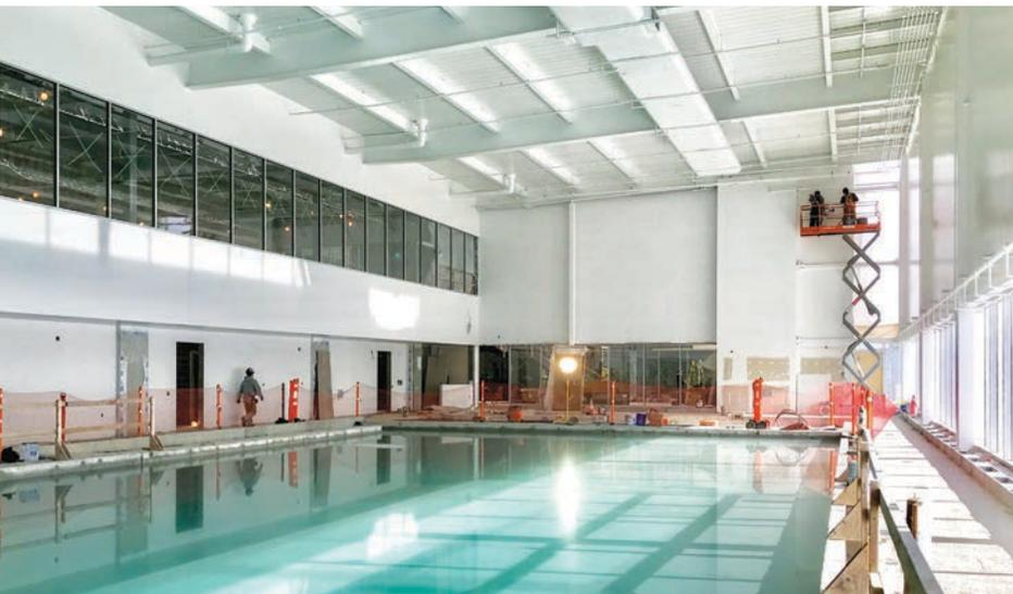
This facility required the fabrication and erection of 585 tonnes of steel comprising of seven 115-foot span AESS trusses, eight girders, and two cantilever trusses each 140-foot long and 22-foot wide, which would be exposed to view in the fitness centre – and which necessitated a full closure of Colborne Street to ensure safe delivery and installation.
