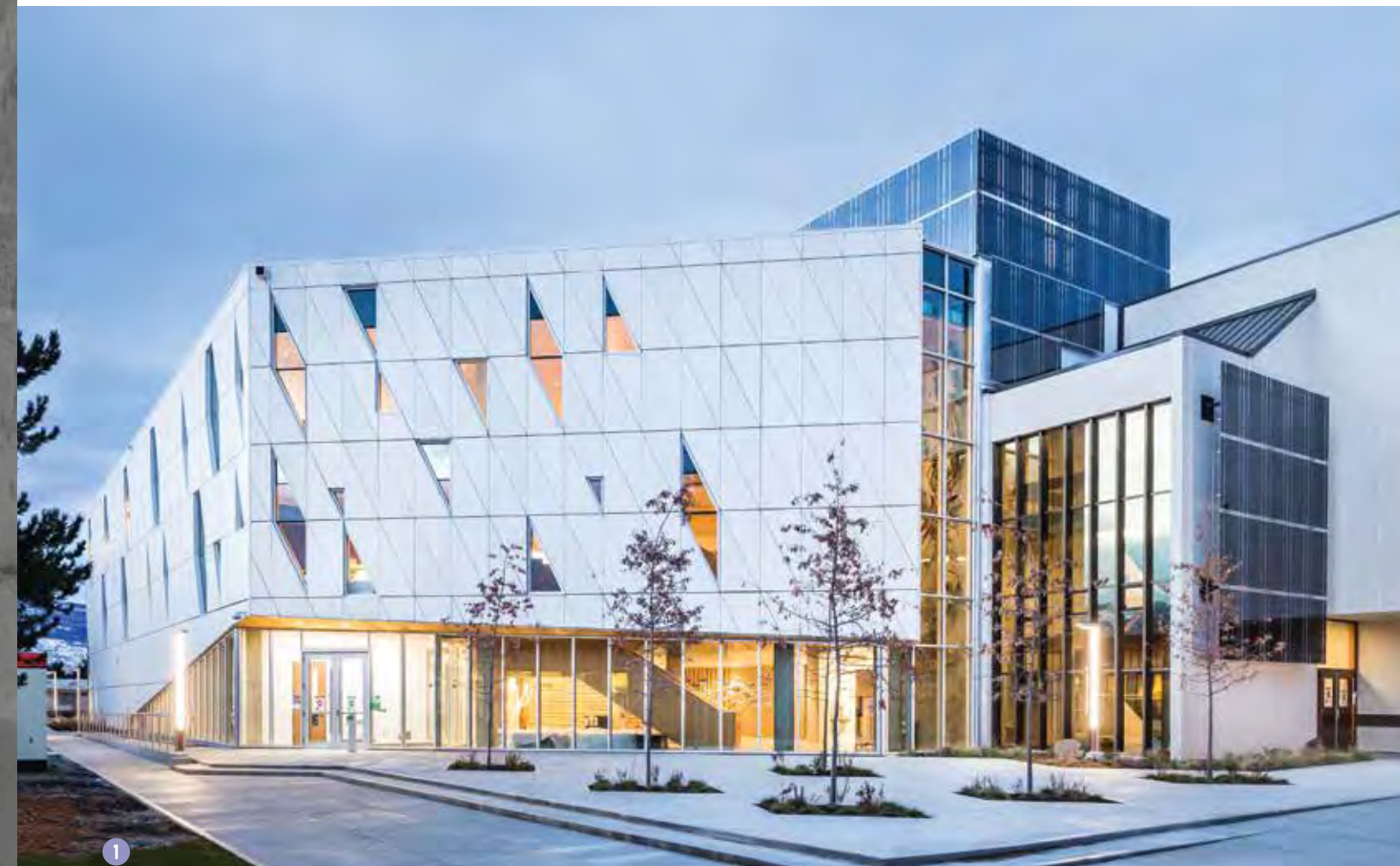
1. The use of waste heat from a wastewater treatment plant, along with integrated photovoltaic panels, means that no gas-fired HVAC systems were required which helped the project to earn the CaGBC's Zero Carbon Building Design certification.
