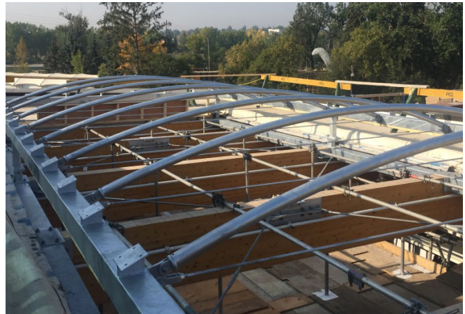
The steel frame structure for the ETFE skylight.
