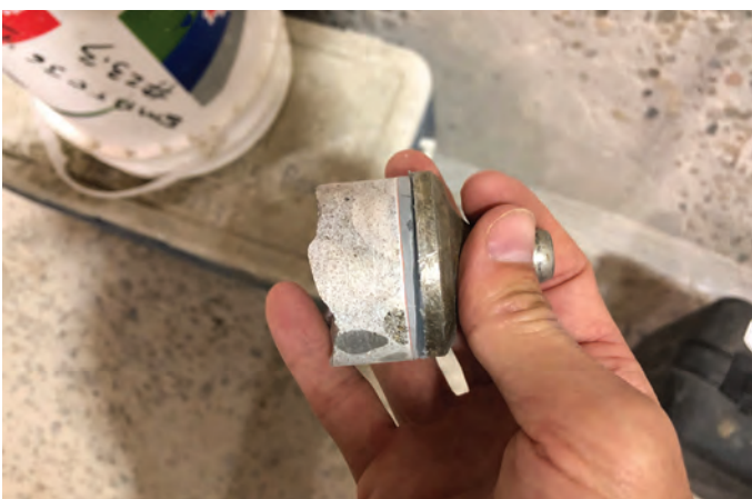
Fig. 6: Failure in original substrate during adhesion strength pull-off testing
