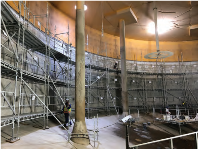
Fig. 4: Access scaffolding set up inside the digester
