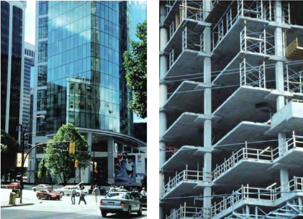
Fig. 1 High rise buildings
