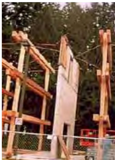
Fig. 5 East Elevation Under Construction
