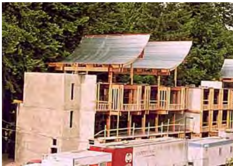
Fig. 6 Southeast Elevation Under Construction
